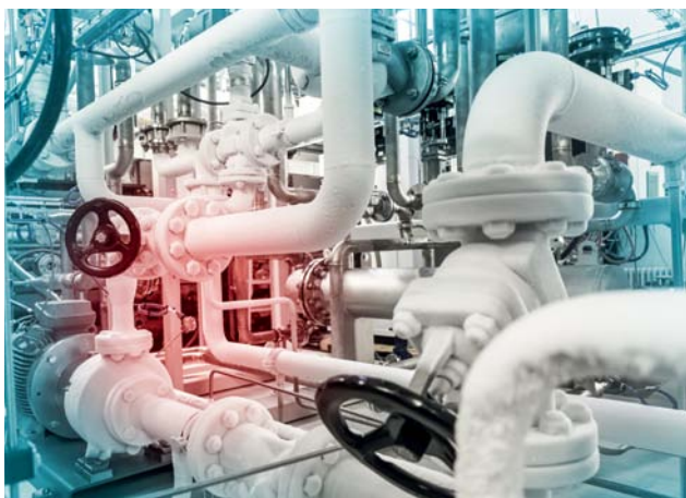
Performance testing during FAT
