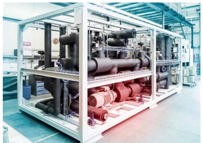
Insulation applied following successful testing
