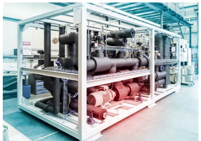
Insulation applied following successful testing
