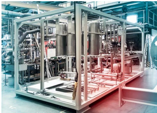
Construction begins once design is frozen
