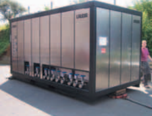
Process cooling unit SUK 600 L in explosion-proof version.
